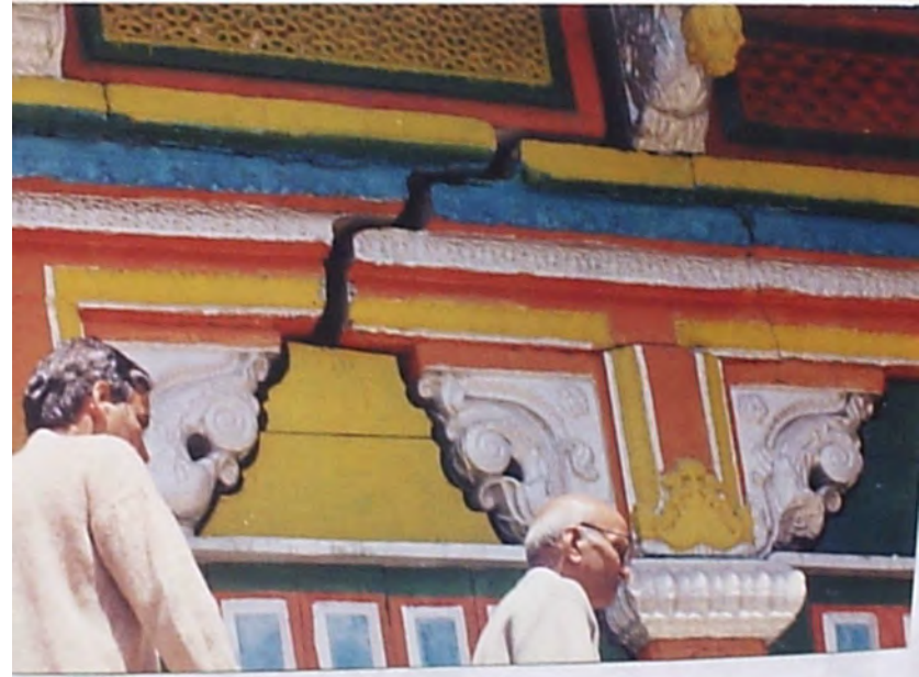
STRUCTURAL CRACKS – BADRINATH TEMPLE FACADE
