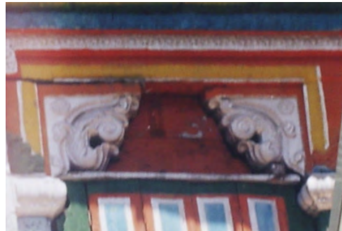
STRUCTURAL CRACKS – BADRINATH TEMPLE FACADE
