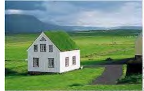
Green roofs have a long tradition, as this farmhouse in a historical park in Iceland shows. David Beattie and his colleagues hope to revive the tradition in Pennsylvania to make roofs that are both beautiful and energy efficient.
